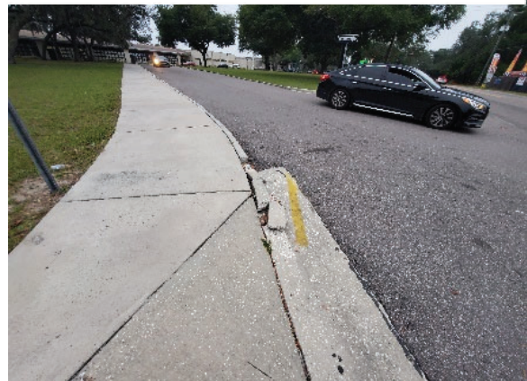
Figure 2-9 - Broken Curb
