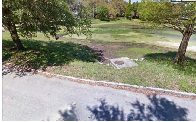
Picture No. 1 - Lake Roberta & Manhole at Outfall Structure
