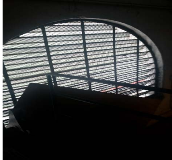
Existing Elevator equipment room grille.
