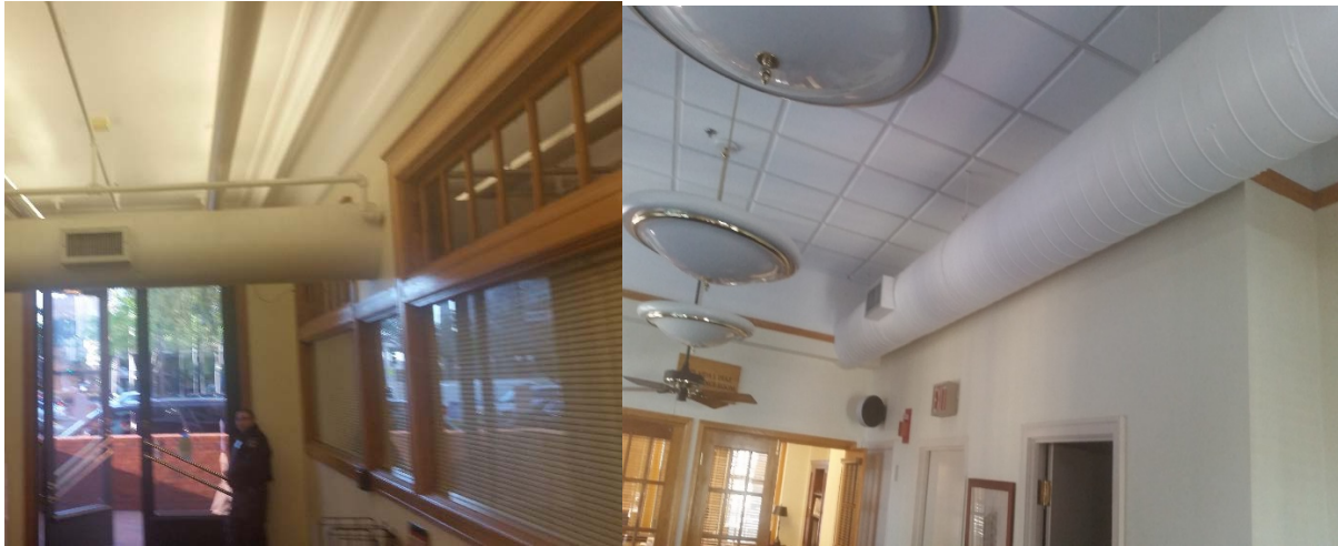
Examples of exposed duct throughout the building.
