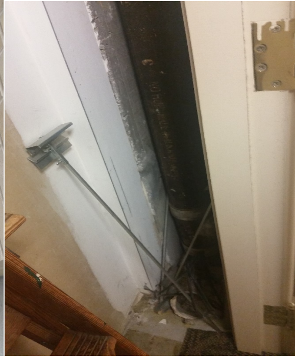
Existing plumbing stack in closet.
