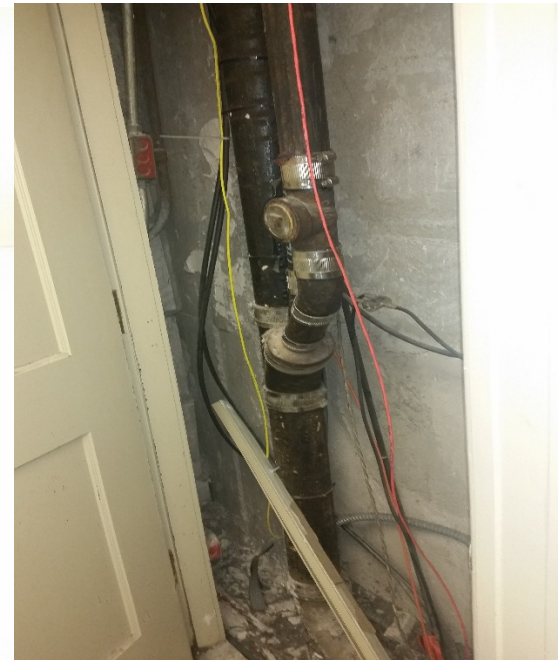
Existing branch stack in closet
