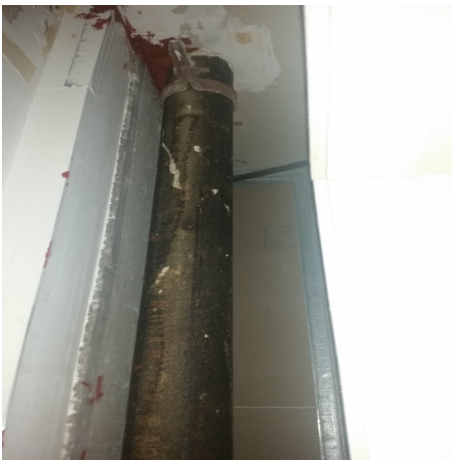
Existing plumbing stack in closet
