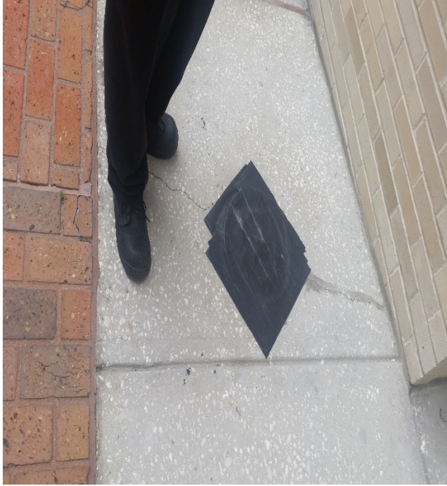
Existing exterior cleanout w/temporary covering
