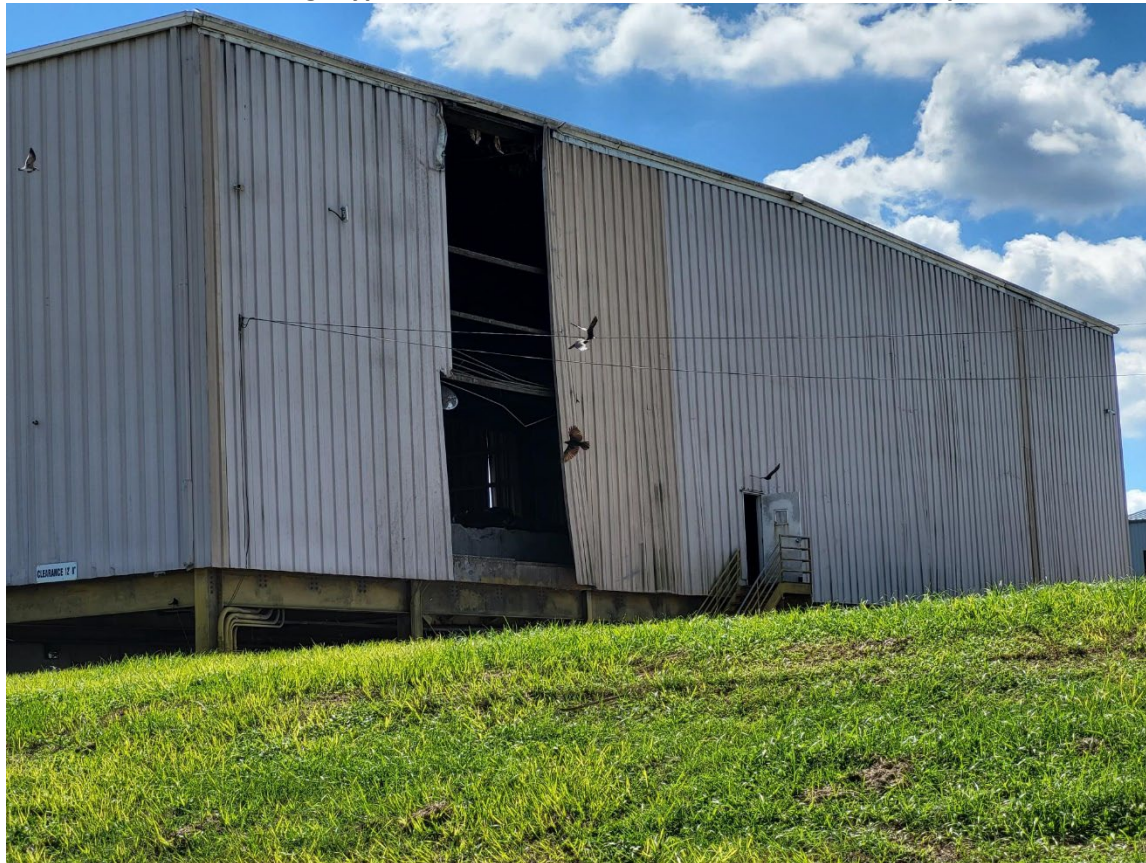
WEST ELEV: Storm damage typ. In various locations, and roof – Assess and Repair
