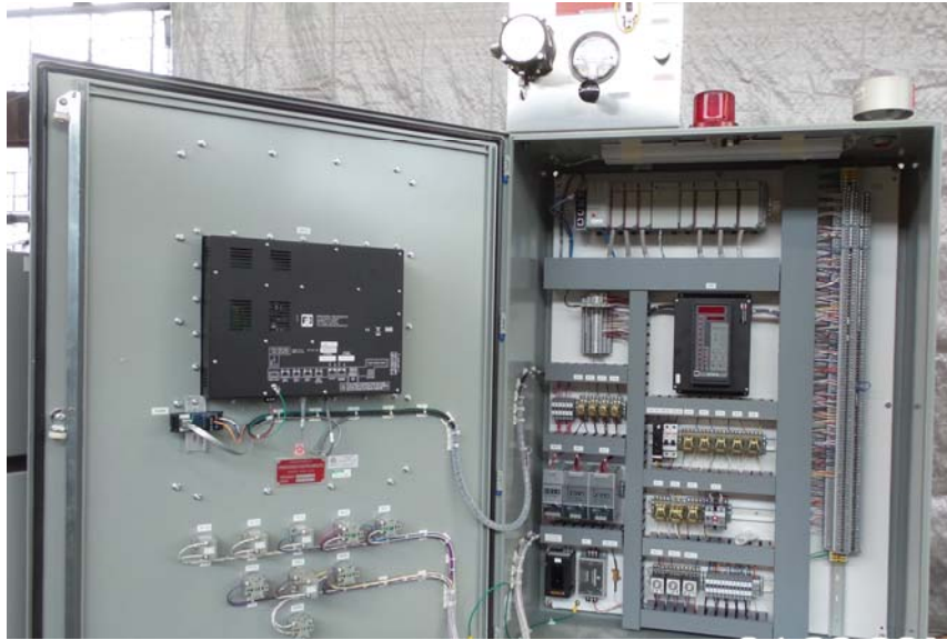
Allen Bradley CompactLogix Based Burner Management System
