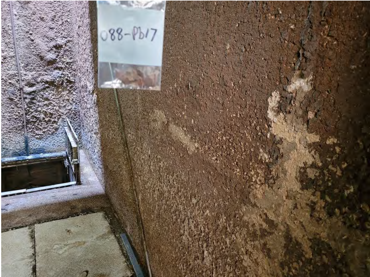
088-PB 17: Beige Paint on Textured Concrete [NLD]
