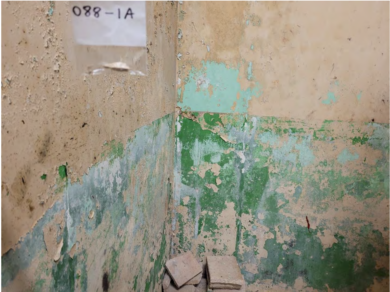
088-1A: Concrete Flooring/Walls [NAD]
