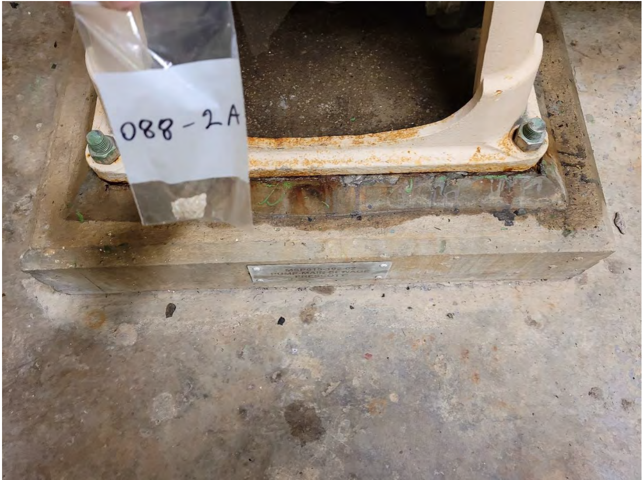
088-2A: Concrete Pedestals [NAD]
