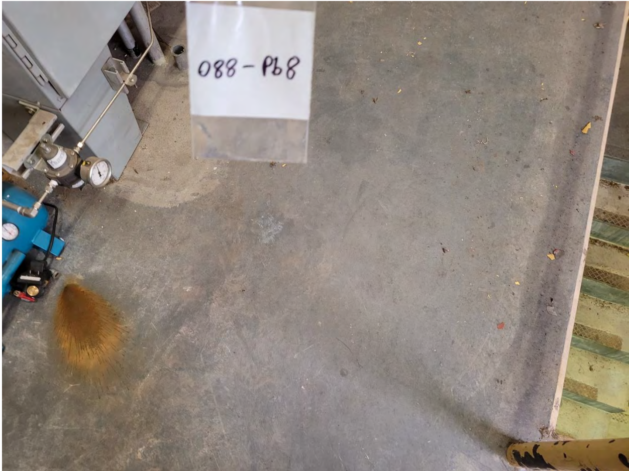
088-PB 8: Grey paint on Concrete Flooring [NLD]
