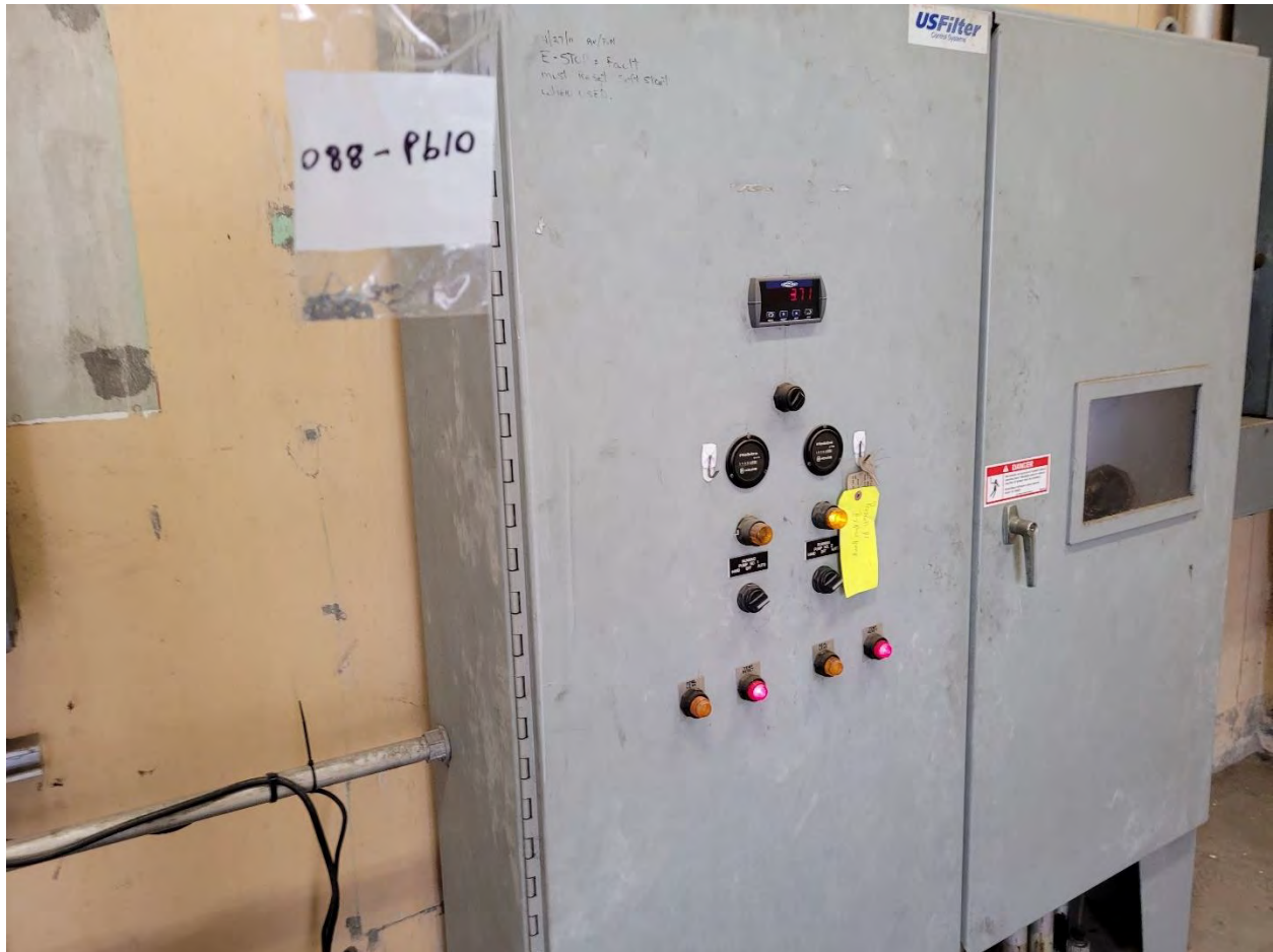
088-PB 10: Light Grey Paint on Metal Cabinets [NLD]
