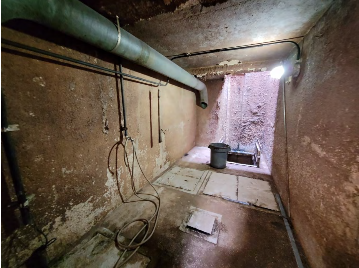
Pumpstation 192: Wet Well, Level 2
