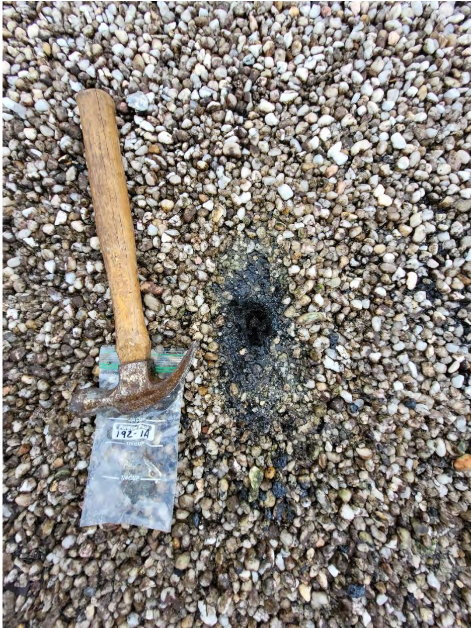
192-1A: Built-up Roof Material [NAD]
