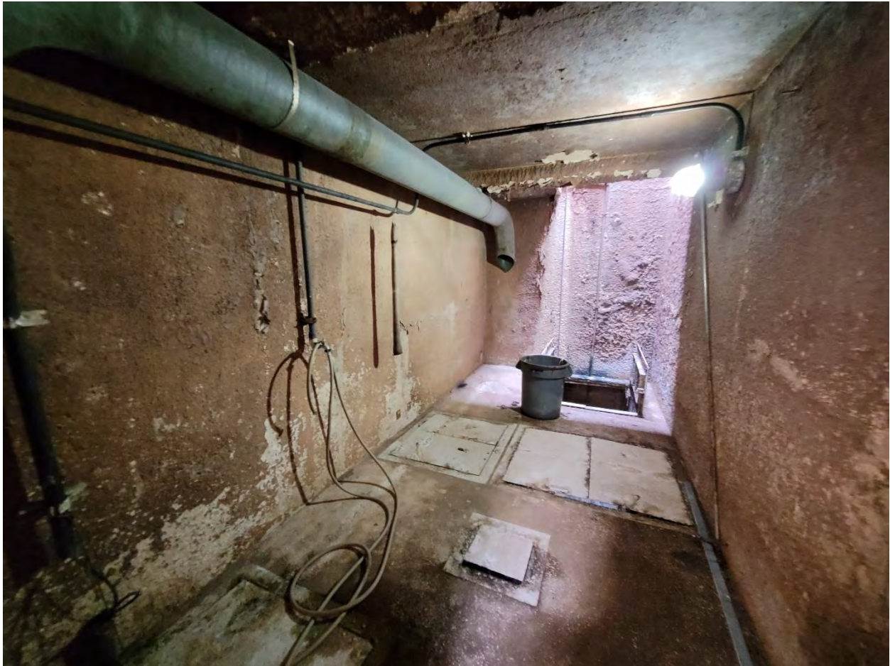
Pumpstation 192: Wet Well, Level 2
