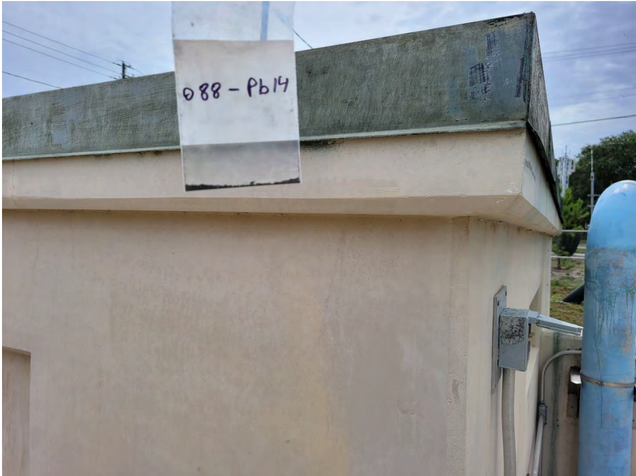
088-PB 14: Grey Paint on Metal Drip Edge [0.060 % wt]
