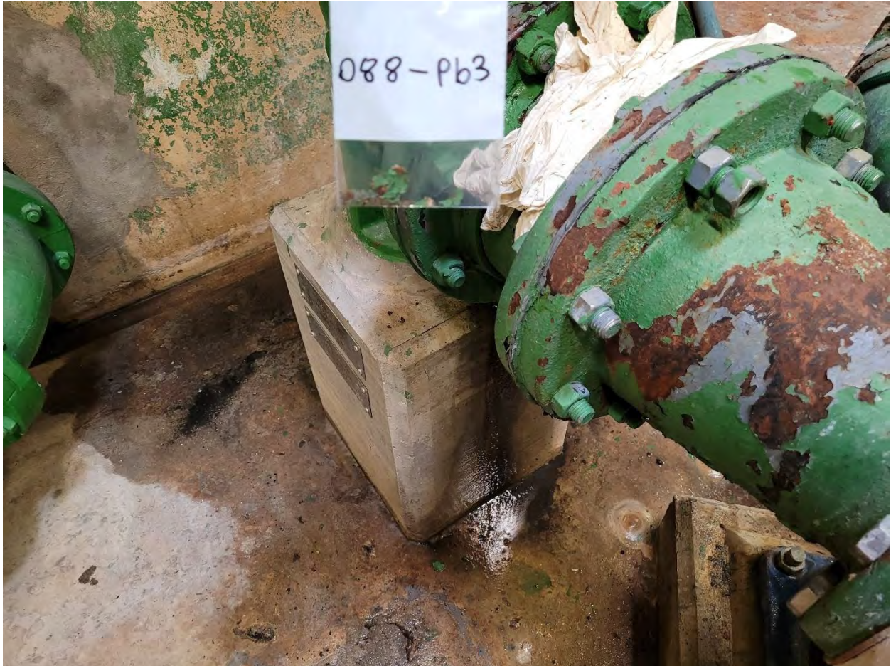
088-PB 3: Green Paint on Metal Pipes [NLD]
