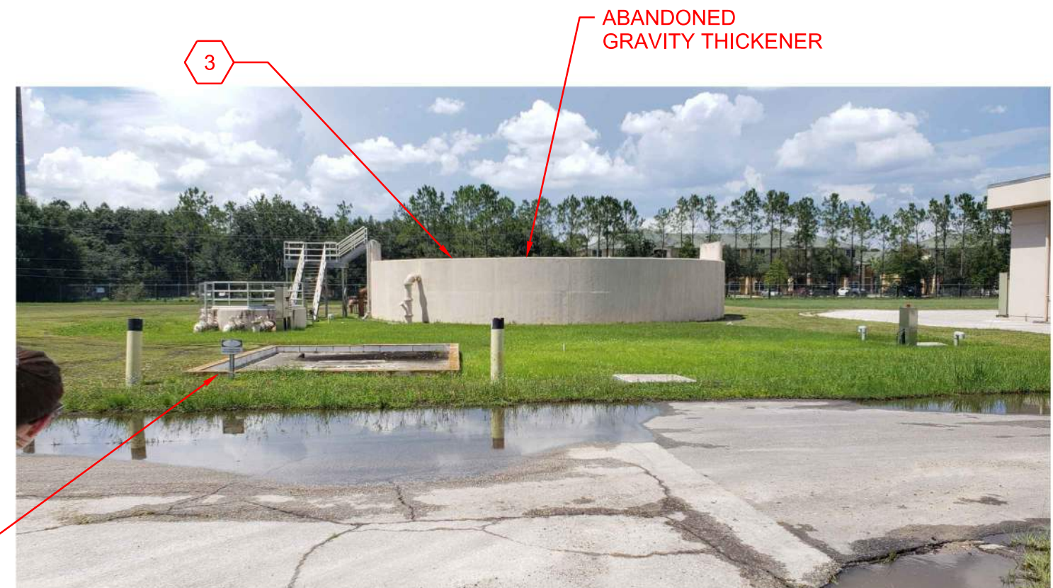
PHOTO DETAIL: GRAVITY THICKENER TANK TO BE DEMOLISHED
