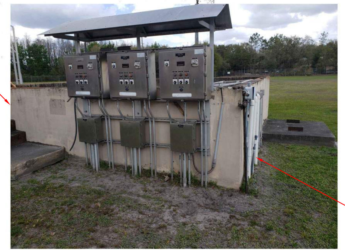
PHOTO DETAIL: CHEMICAL CONTAINMENT AREA TO BE DEMOLISHED
