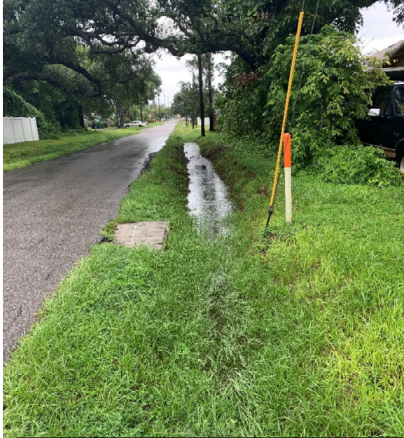
LOCATION: W. CHERRY ST. LOOKING SOUTH EXISTING SWALE WITH UNSAFE SLOPES
