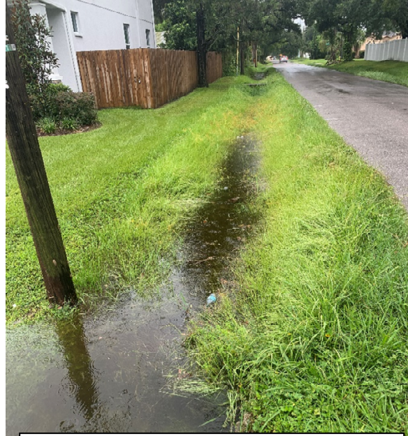
LOCATION: W. PALMETTO ST. LOOKING SOUTH EXISTING SWALE WITH UNSAFE SLOPES
