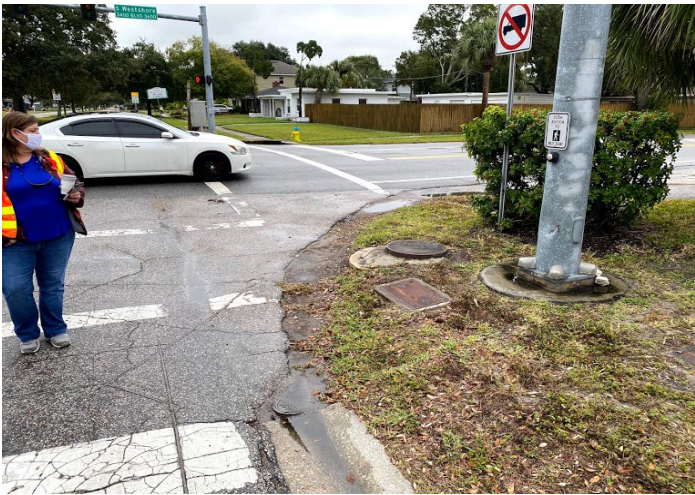
Figure 9: Inaccessible push buttons at West Shore Blvd. and Dale Mabry Hwy, left and right, respectively
