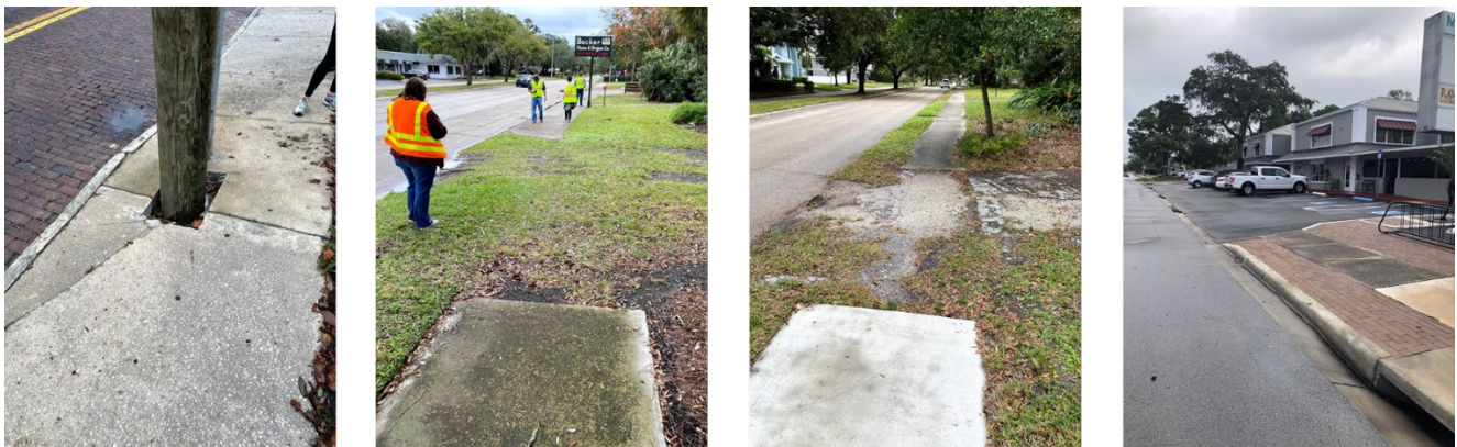
Figure 7: Sidewalk gaps, drop-offs, and lack of delineation through wide driveways are some of the hazards and accessibility obstacles observed.
