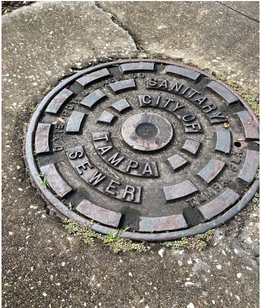
Figure 8: Drainage inlet within sidewalk in area of sidewalk swale (left); sanitary sewer manhole cover within southside sidewalks (right)
