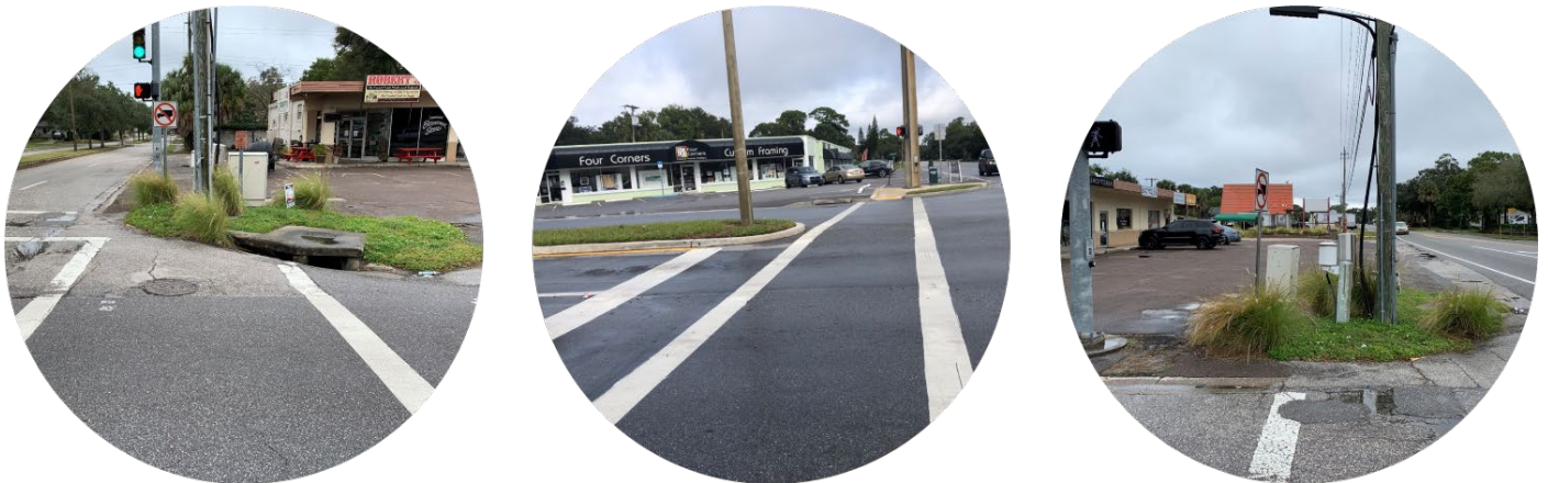
Figure 12: Long crossing distances for pedestrians and lack of ramps and landings make intersections dangerous and inaccessible.
