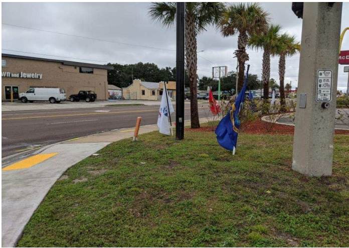
Figure 9: Inaccessible push buttons at West Shore Blvd. and Dale Mabry Hwy, left and right, respectively
