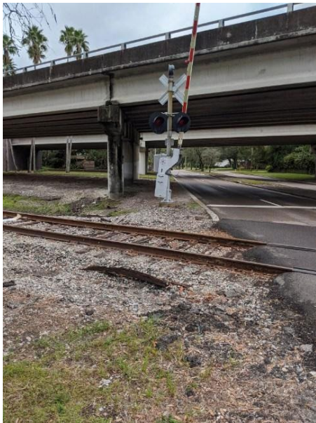
Figure 10: CSX Rail crossing with no sidewalk on north side
