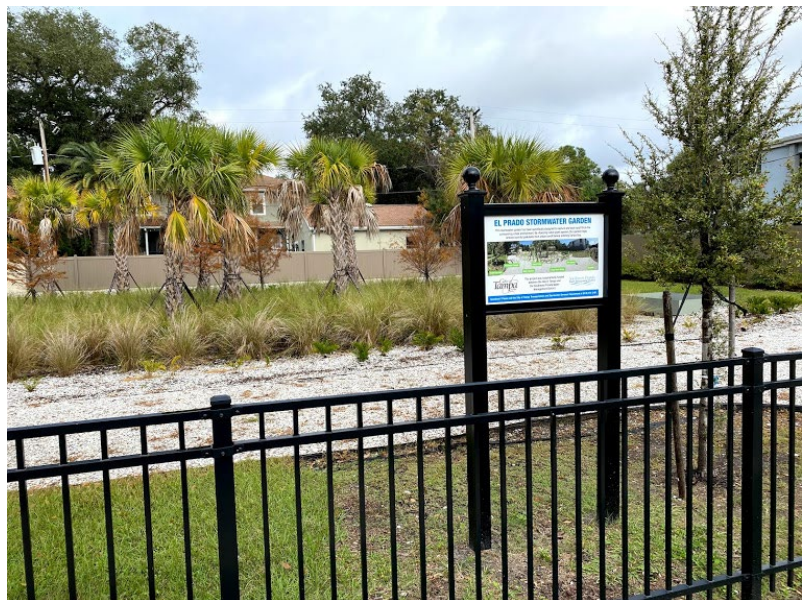
Figure 11: Existing El Prado Stormwater Pond
