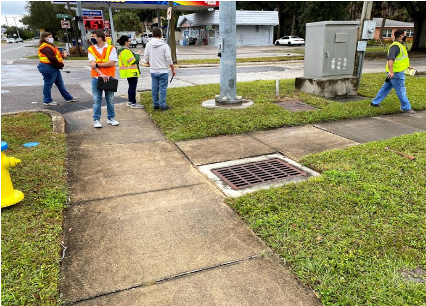
Figure 8: Drainage inlet within sidewalk in area of sidewalk swale (left); sanitary sewer manhole cover within southside sidewalks (right)
