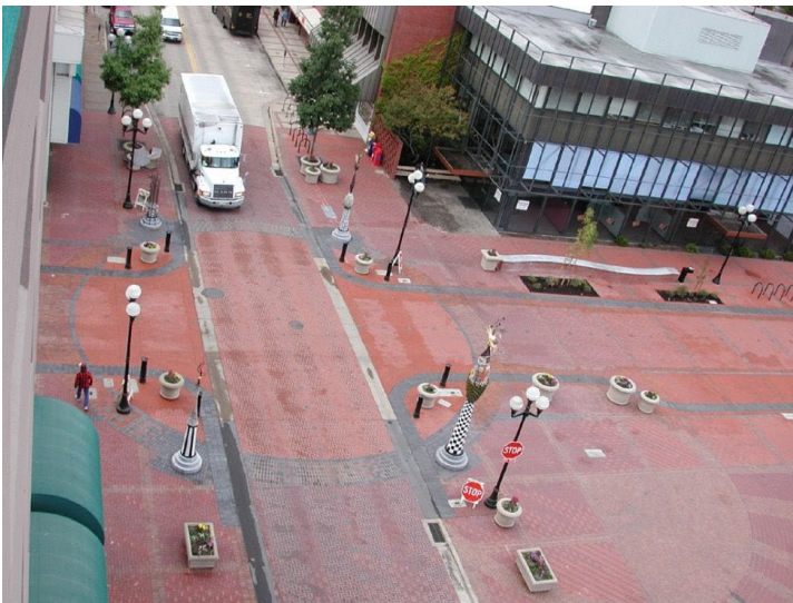
Figure 3 Example of a Raised Intersection | National Association of City Transportation Officials (NACTO)
