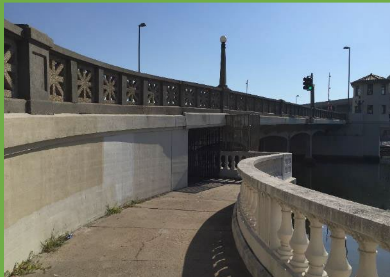
Southwest side of the Platt St. Bridge.
