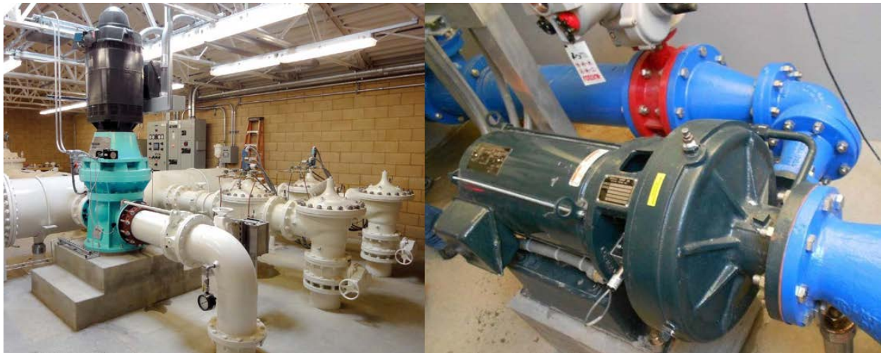
Figure 13 – Francis Turbine (Canyon Hydro, left) and PAT (Rentricity, right).
