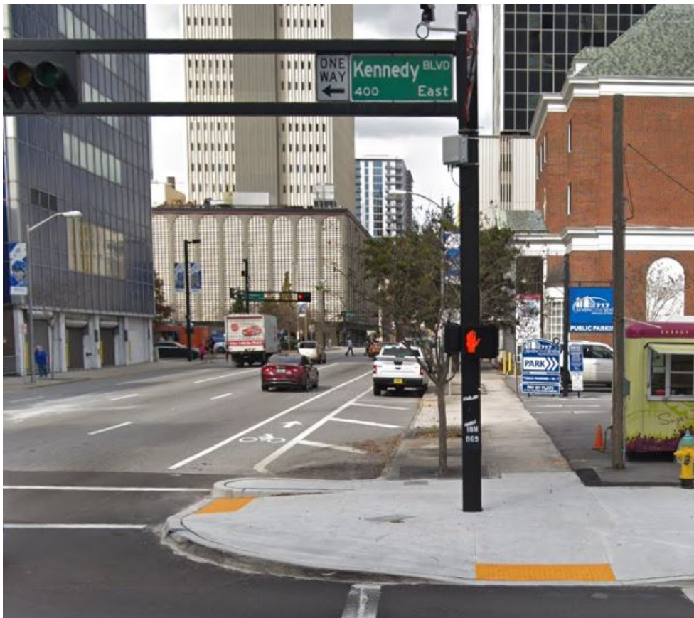
Figure 27. Example of Curb Ramps Along Extension Corridor
