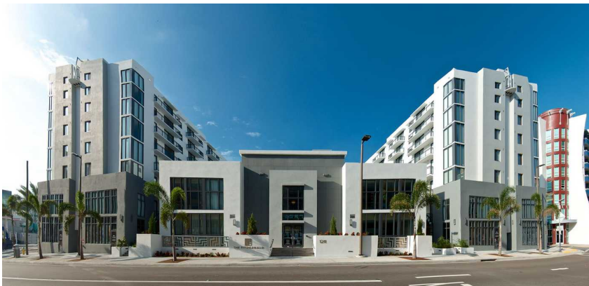
Figure 8. The Fitzgerald (Mixed-Use Residential), Located 0.10 miles from the existing Tampa Streetcar alignment
