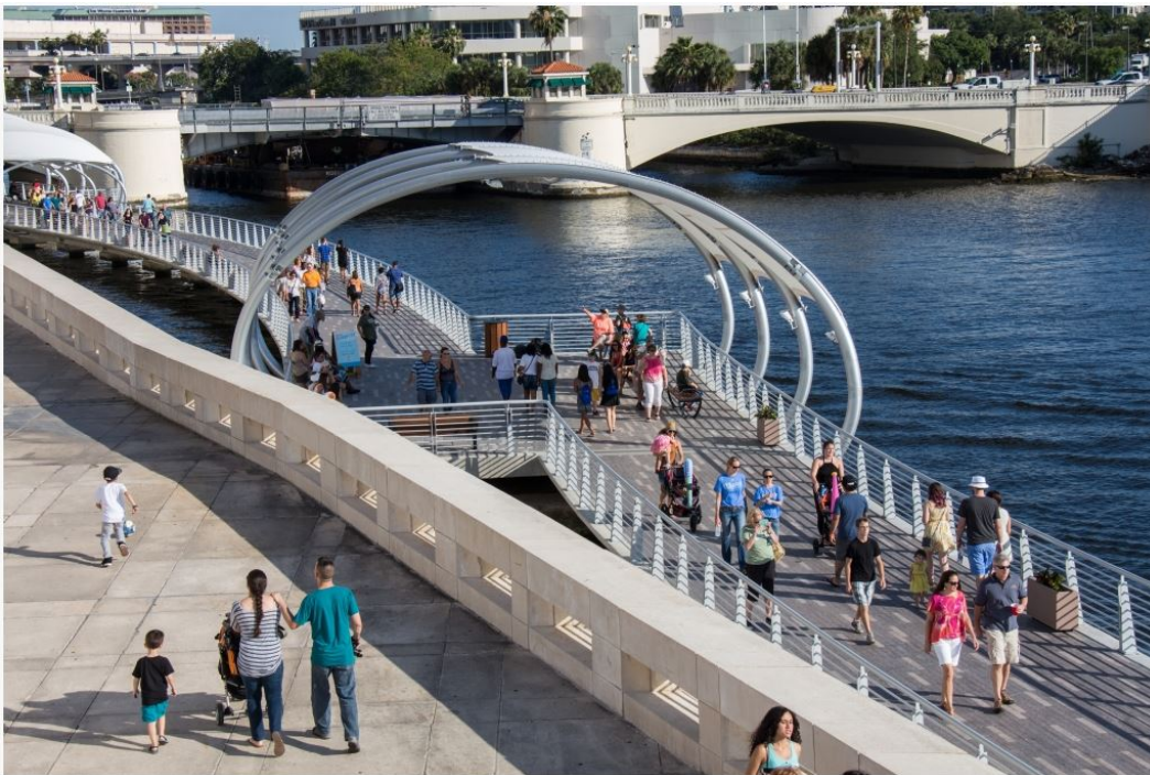
Figure 28. The Tampa Riverwalk
