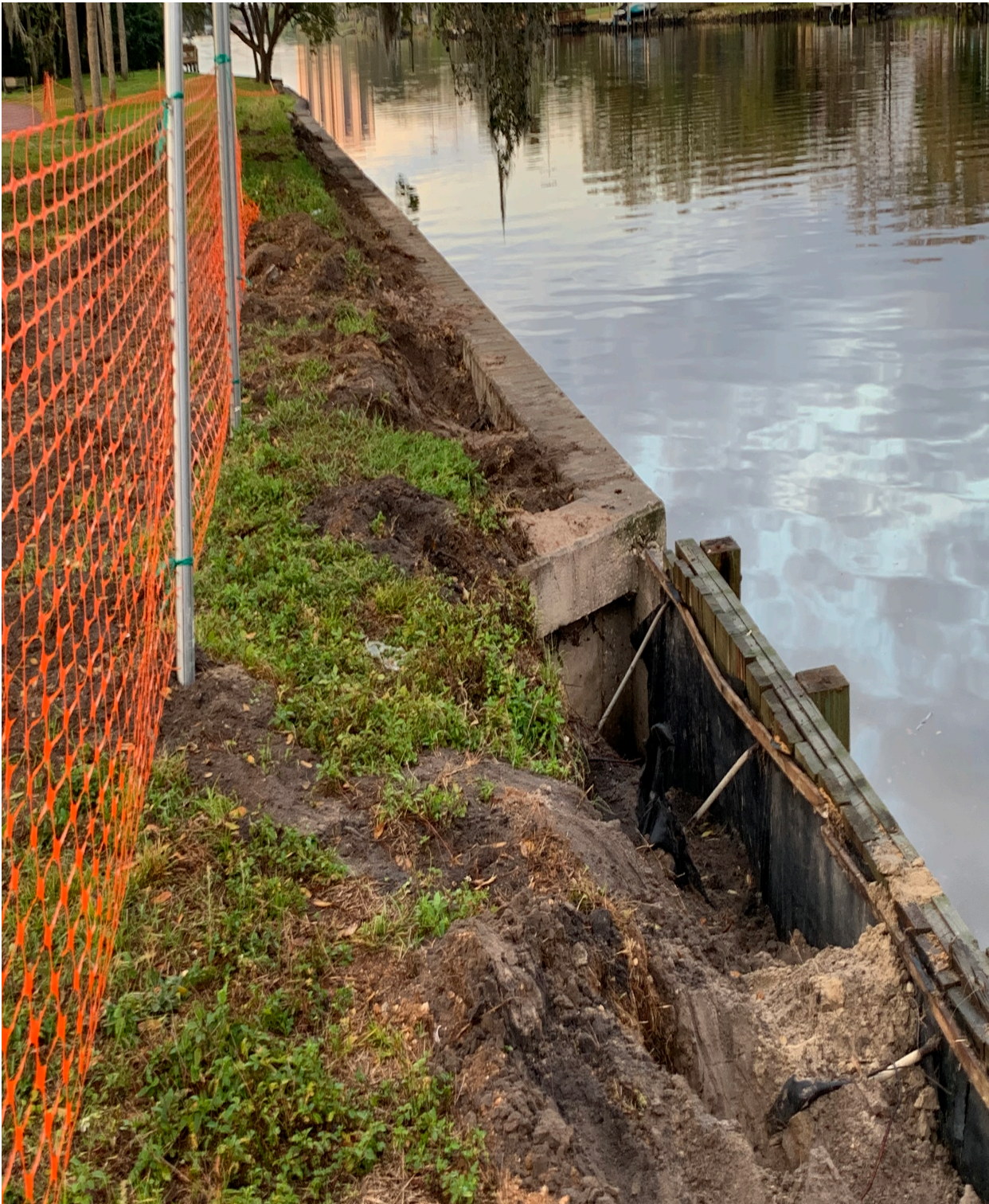
EXHIBIT D: EXISTING WOODEN SEAWALL
