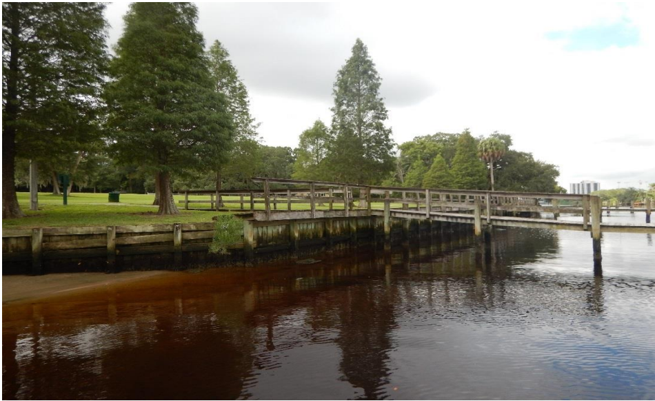
Photo 9-1. Timber boardwalk and retaining wall at Rivercrest Park
