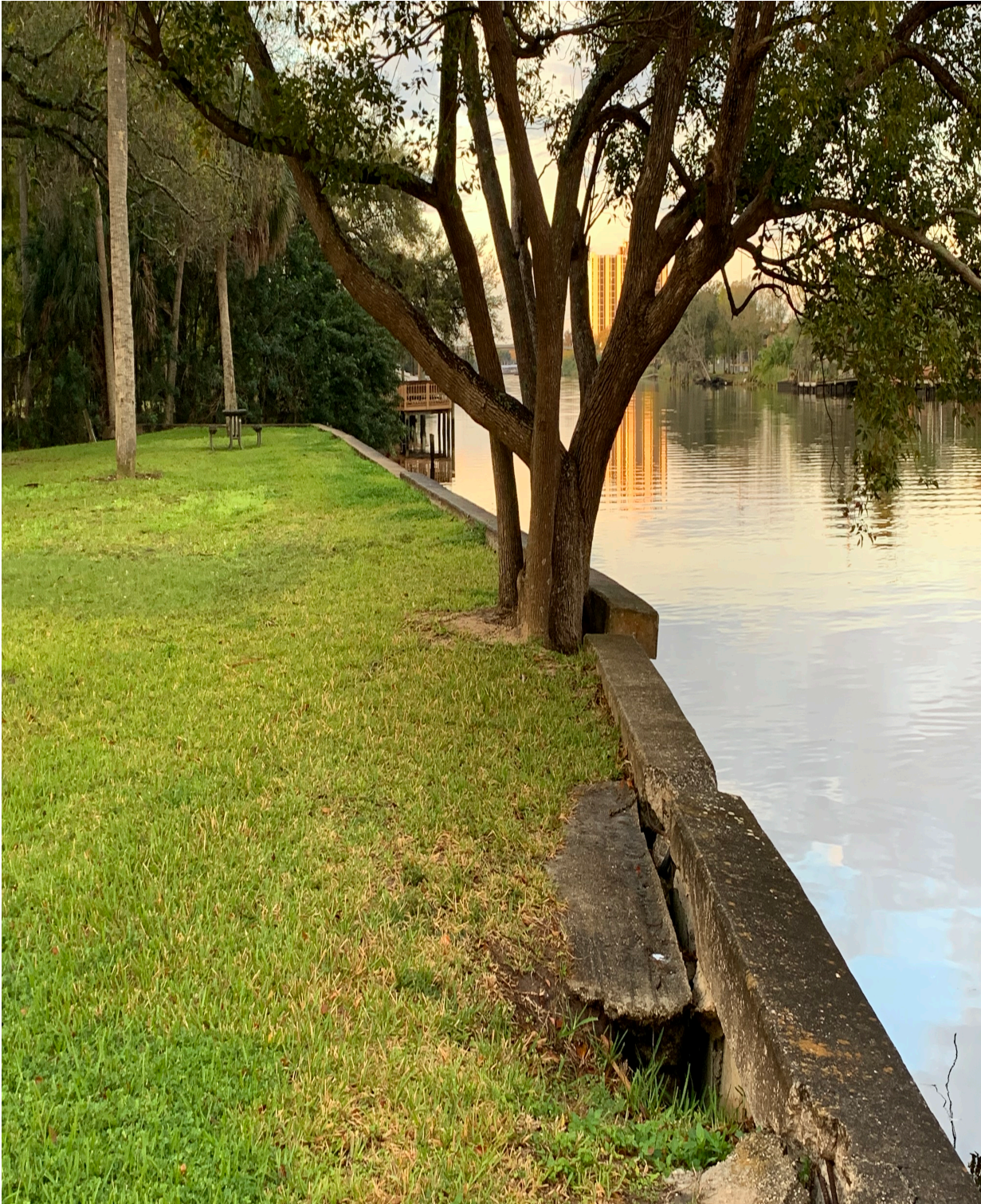
EXHIBIT F: EXISTING CONCRETE SEAWALL
