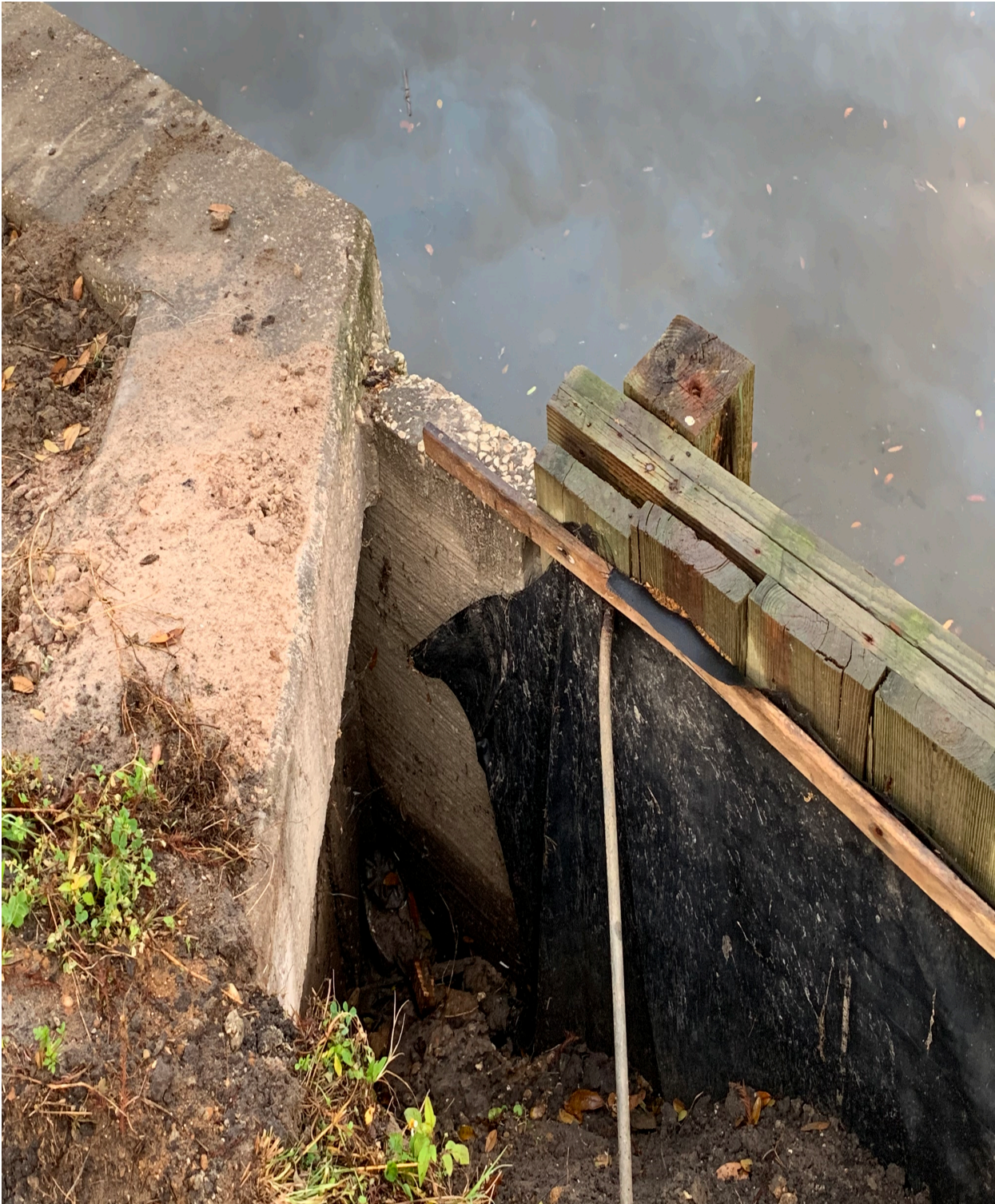
EXHIBIT E: EXISTING WOODEN SEAWALL AT TRANSITION TO CONCRETE
