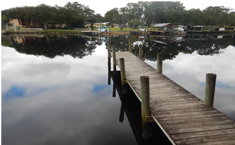
Photo 9-9. Typical conditions observed at Dock 4
