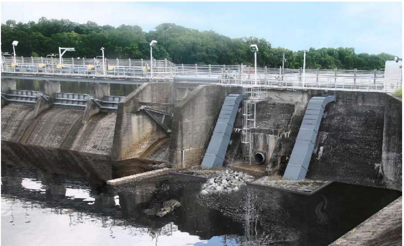
Dual Siphon (Downstream View) at Vertical, Non-spillway Section of Dam
