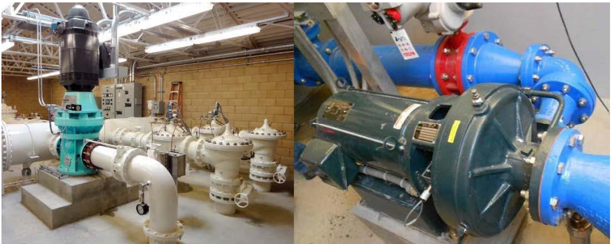
Francis Turbine (Left) and Pump as Turbine (Right) Examples
