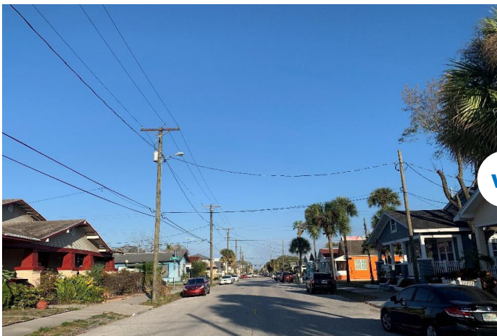
Typical neighborhood power lines in Tampa
