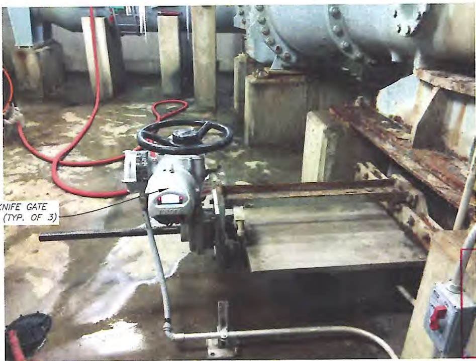
PROPOSED CONFIGURATION FOR KNIFE GATE VALVE ACTUATORS
